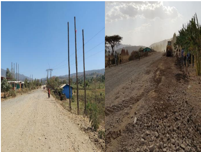
Figure 1: Initial Phases of Gravel Road Construction for C1 & C2
